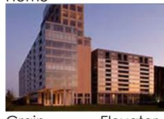
Grain Apartment Elevator
